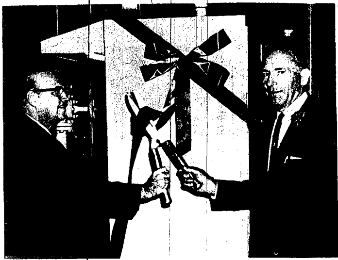
RIBBON CUTTING at the new Norbert Brugger addition to the Wayne power plant was performed by Mayor William Koeber (left) and Norb Brugger, in whose honor the new structure has been named. Former Mayor Chris Tietgen and Councilmen E. G. Smith and Jack Kingston had parts in the open house ceremony Thursday.
